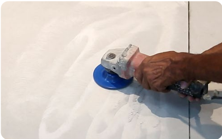
STEP 1 : GRINDING
