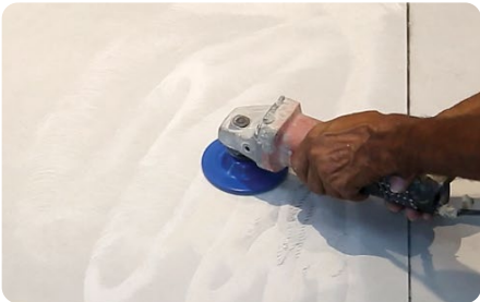
STEP 1 : GRINDING
